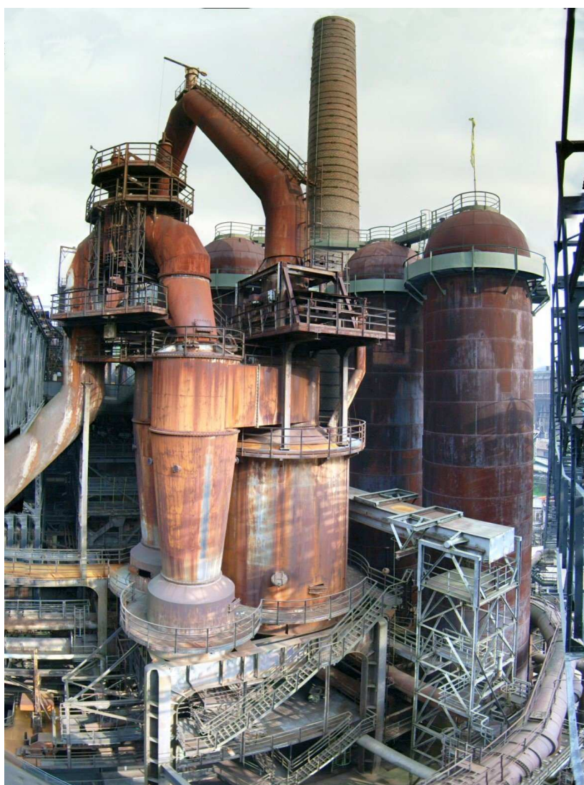
Figure 9.3.1.: Ironworks in Völklingen, Germany (UNESCO World Heritage Site since 1994), as an example for two different kinds of solid-gas reactions, iron ore smelting (reaction of iron oxides with gaseous carbon monoxide; when operating \leq 1986 ) and corrosion of steel in air (after closing in 1986); By Lokilech - Own work, CC BY-SA 3.0, https://commons.wikimedia.org/w/index.php?curid=1331378 , download August 8, 2017.
